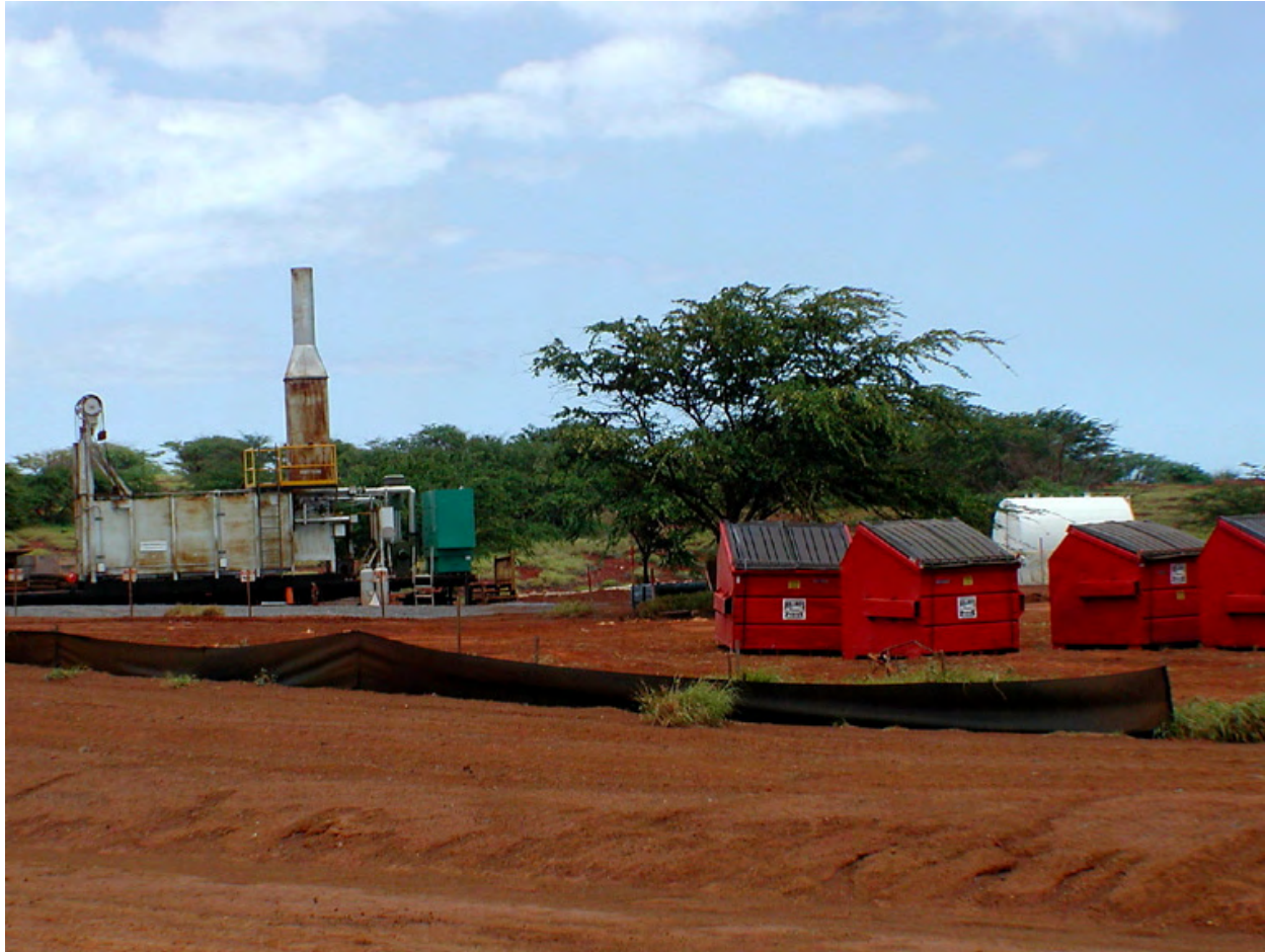
Figure 6: Thermal Processing Unit (TPU)
